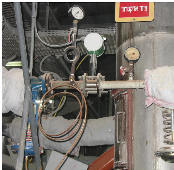
*An inline wafer multivariable steam meter is used to measure and control steam at an animal food plant in Israel. The steam is injected into the dry pellets to give them constancy and uniformity.*
