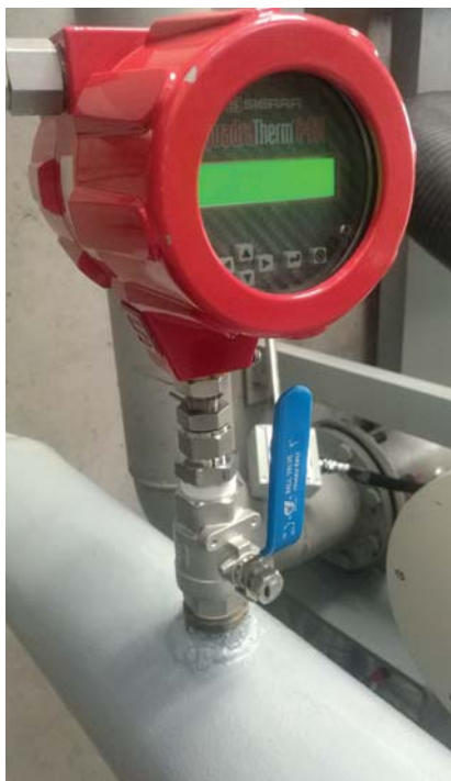
A closer look at the thermal mass flowmeter
