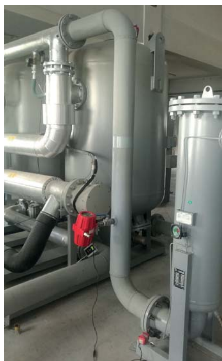
A thermal mass flowmeter measuring compressed air
