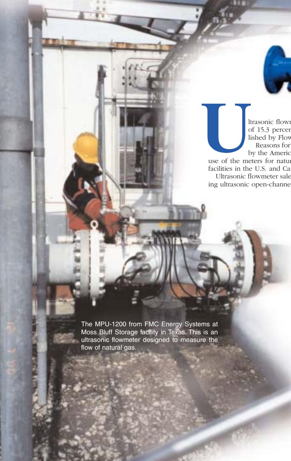
The MPU-1200 from FMC Energy Systems at Moss Bluff Storage facility in Texas. This is an ultrasonic flowmeter designed to measure the flow of natural gas.
