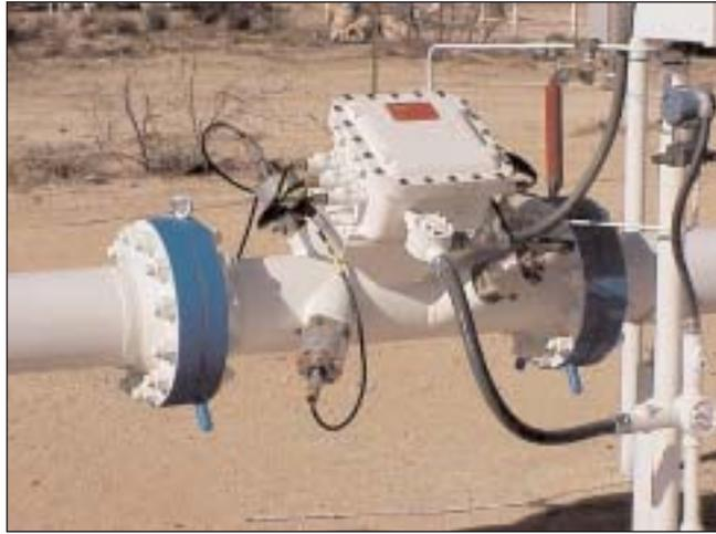
An 8-inch Q.Sonic flowmeter from Instromet, designed to measure natural gas flow.
