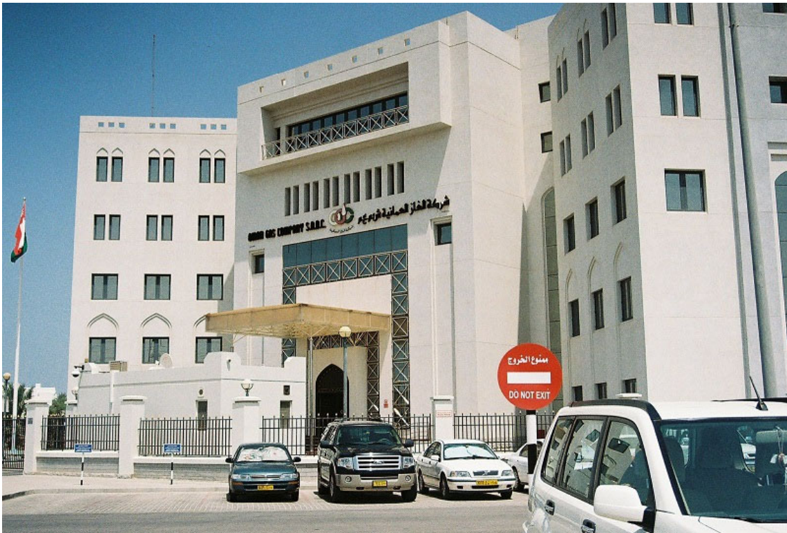
Oman Gas Company (Photo by Flow Research)
