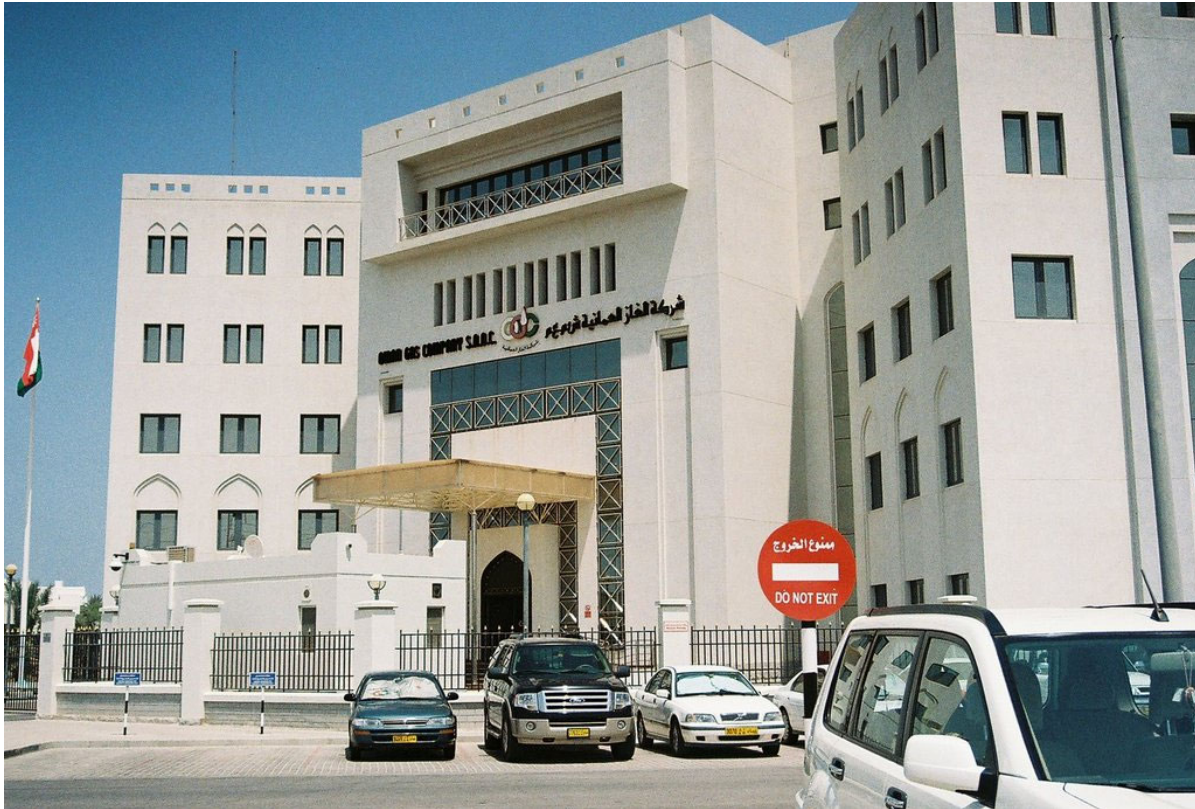
Oman Gas Company Photo by Flow Research
